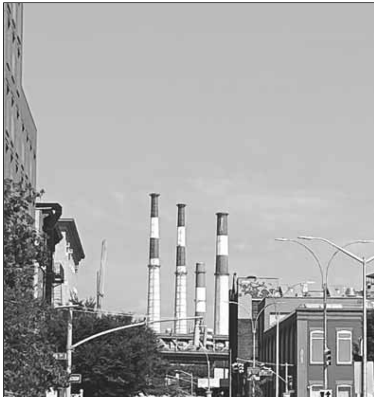
The Ravenswood "peaker" plant in Queens.
